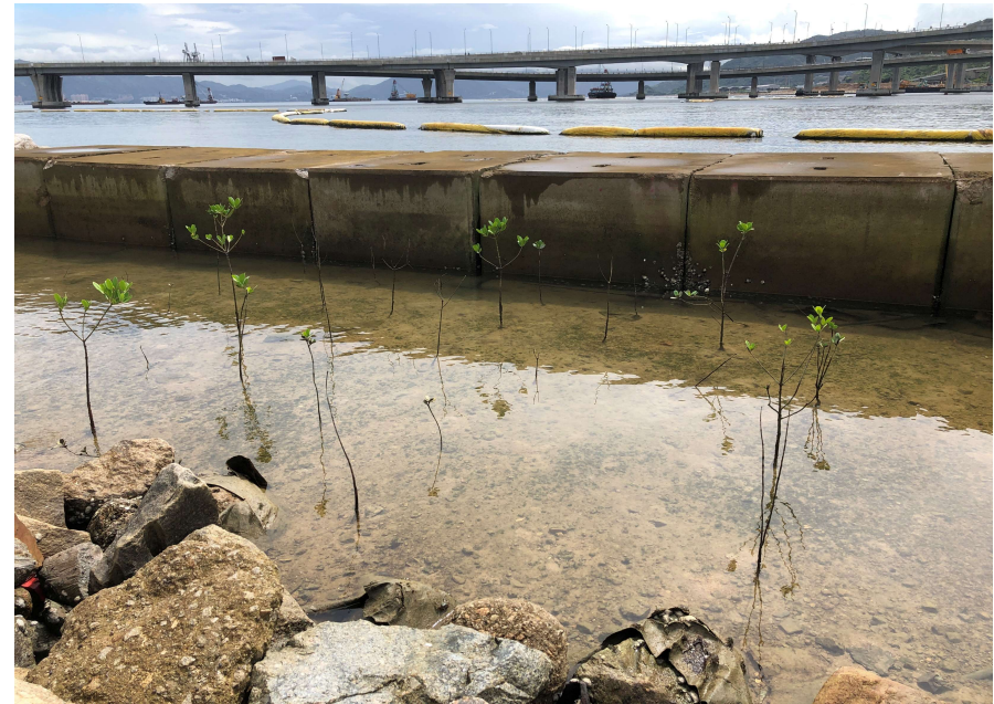
General View of Mangrove Eco-shoreline Lower Terrace
