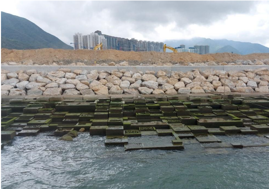
Photo 4 – Natural Rock Material/Planting for Artificial Seawall
